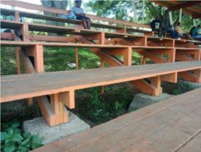
Photo 7: view of northern grandstand footings
