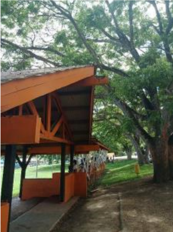
Photo 10: central grandstand ridge beam rotted (at end)
