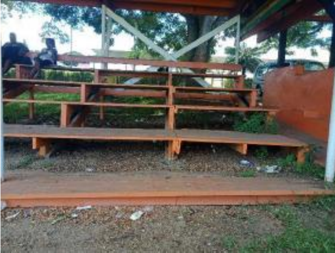
Photo 1: showing damage to end support of seating
