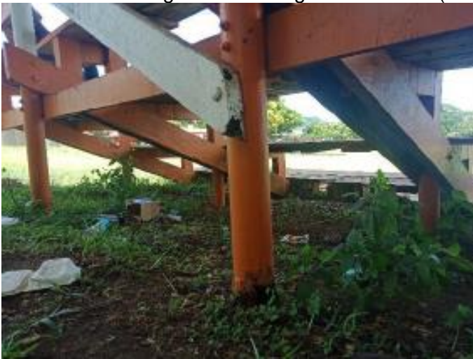
Photo 11: example of steel column rusted at ground level – will have to be cut out and new steel attached/installed
