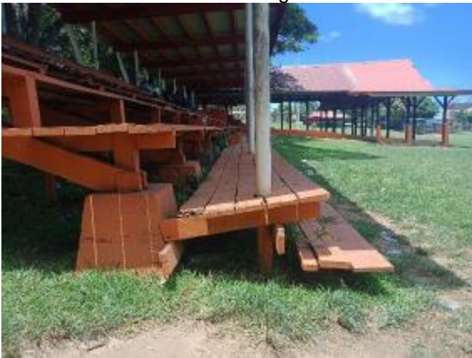
Photo 5: fixing with concrete footing is damaged
