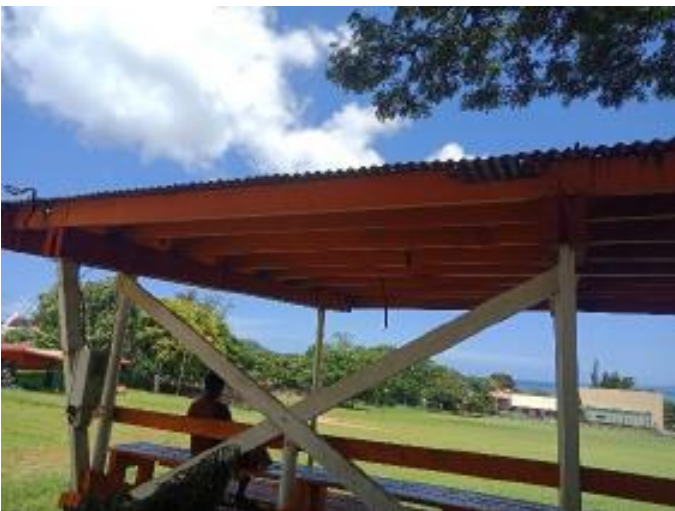
Photo 9: example of damaged timber purlin
