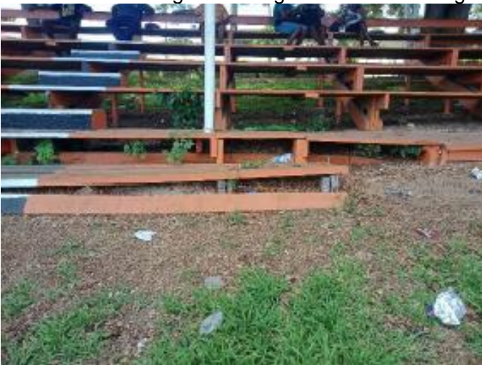
Photo 3: damage to seating structure – northern side
