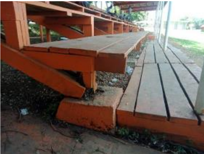
Photo 8: example of rotted timber seating supported
